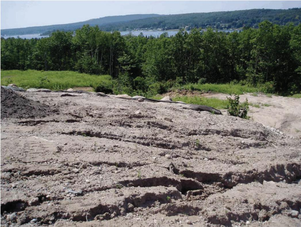
**Photograph 9. Construction activity to southeast of property, showing erosion and sediment released towards property (August 9, 2010).**
