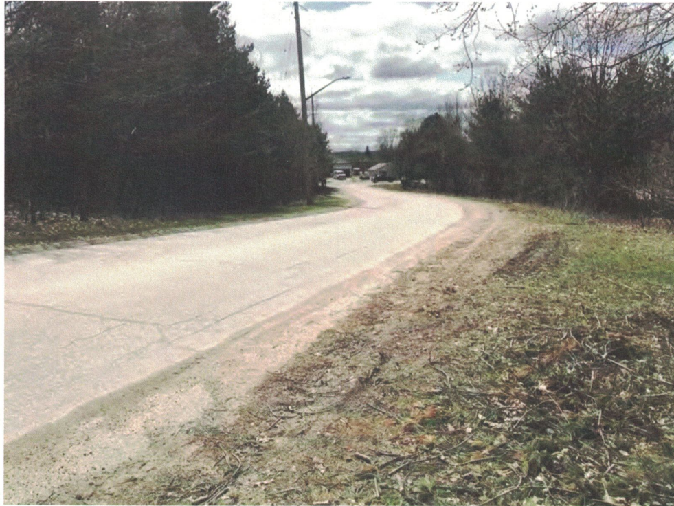
Plate B19: West Forest Area Field Conditions as seen from LeCarron; looking south
