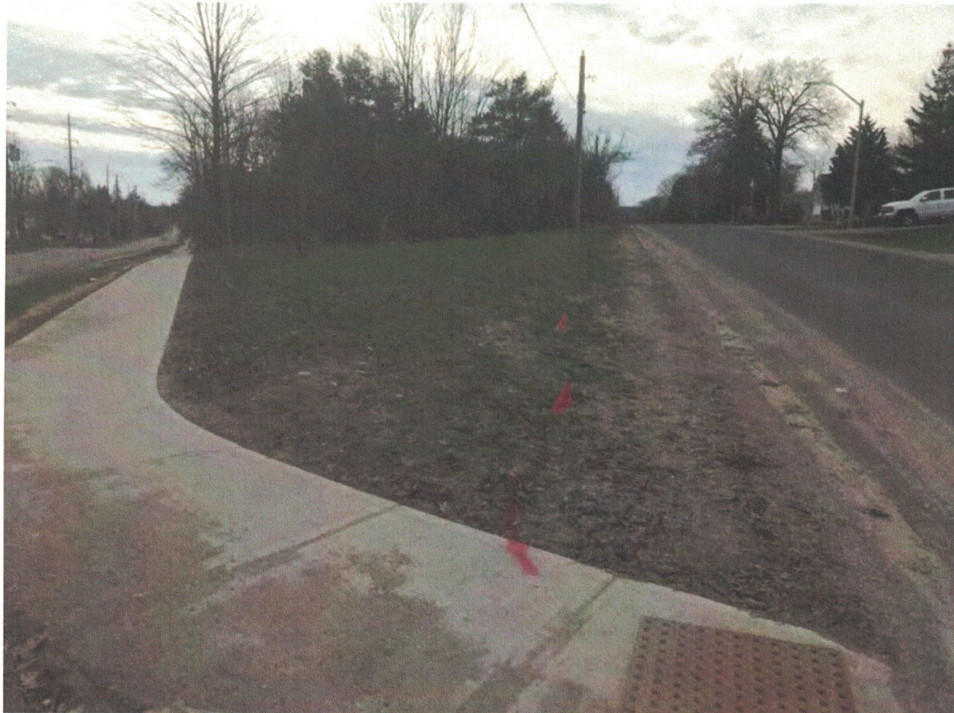
Plate B24: East End of Property Field Conditions; looking west along Burke & Robert
