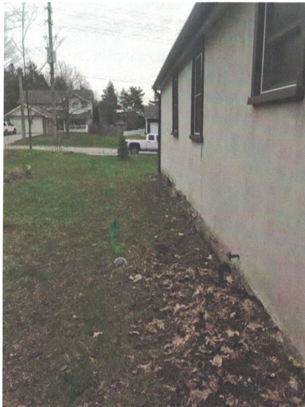
Plate B11: Field Conditions & Utility Location Markers at East Side of Property; looking south
