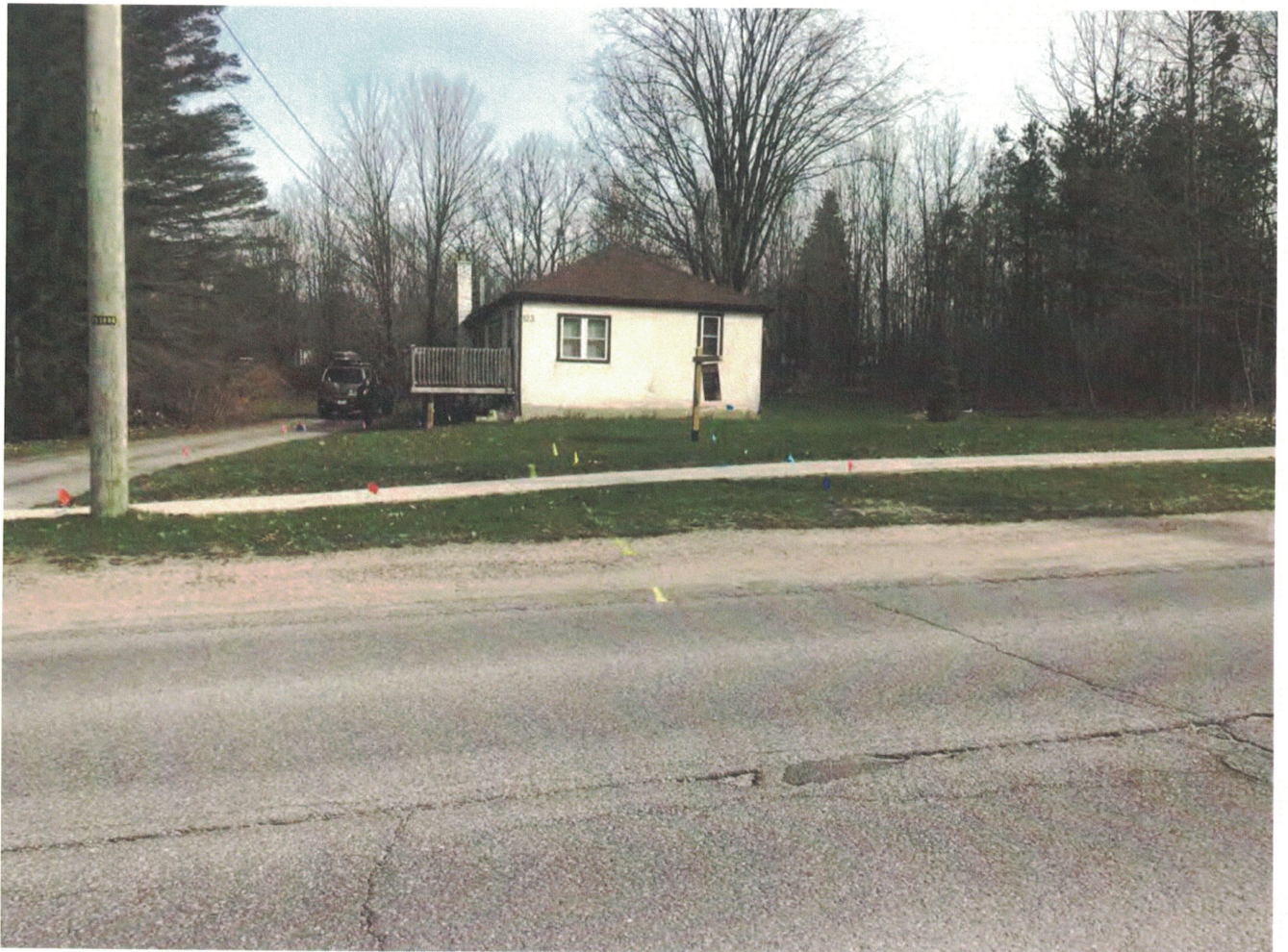
Plate B2: Utility Location Markers at Front of Property; looking north
